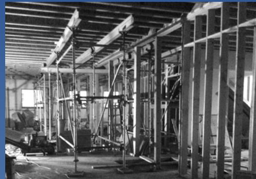
Over at the new Welcome Center site, where district offices also will be located, new concrete footings and foundations have been poured. Also support trusses on the second floor have been installed in preparation for a new roof beam. In March, we expect to see a new roof on the building.
